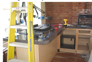
With the cabinets in place, the wiring will now begin.
